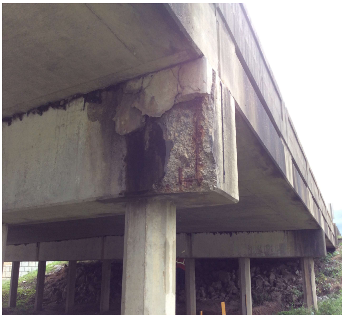
PHOTO 1 Description Spalls with rebar exposed to Left end of cap @ Bent 2.
