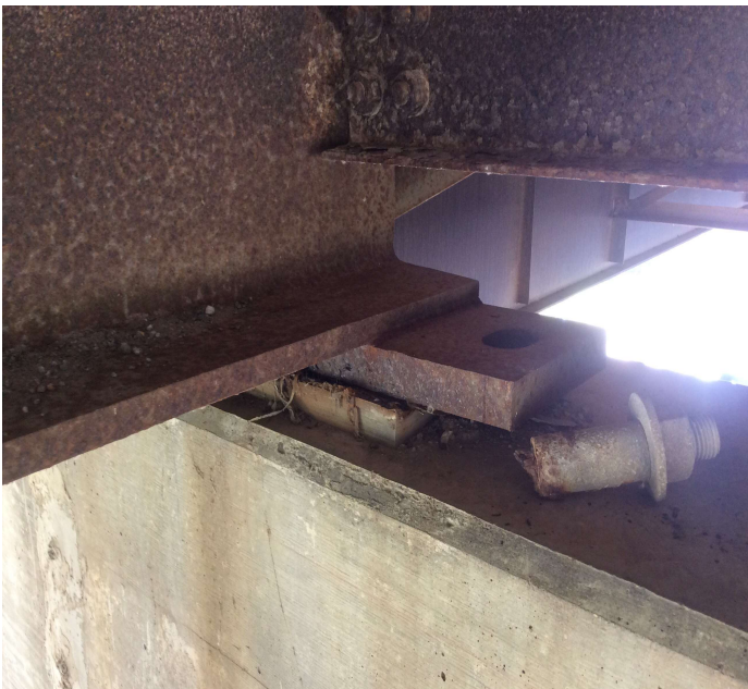
PHOTO 1 Description Bearing at Girder 3 Span 18 has broke anchor bolt.
