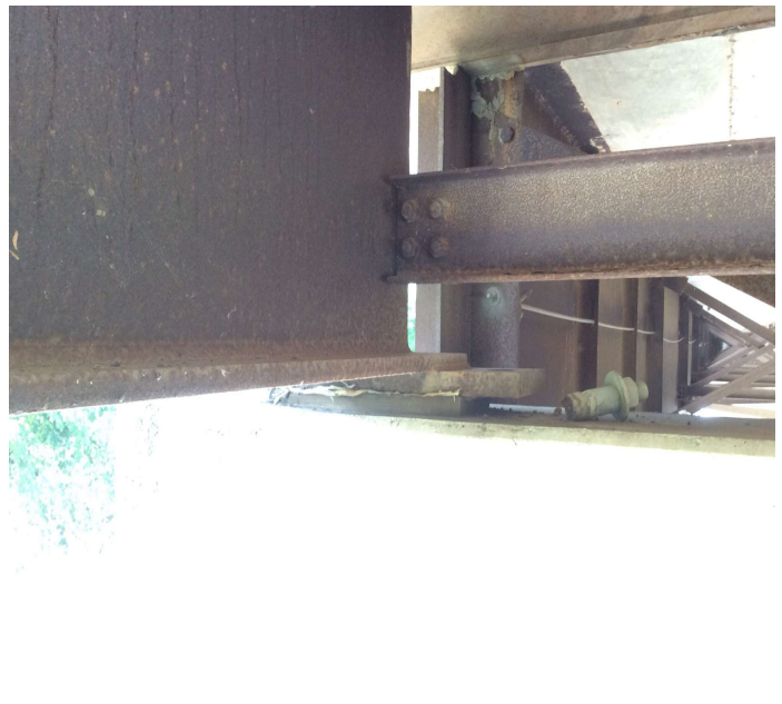
PHOTO 2 Description Bearing @ Girder 1 Span 18 has broke anchor bolt.
