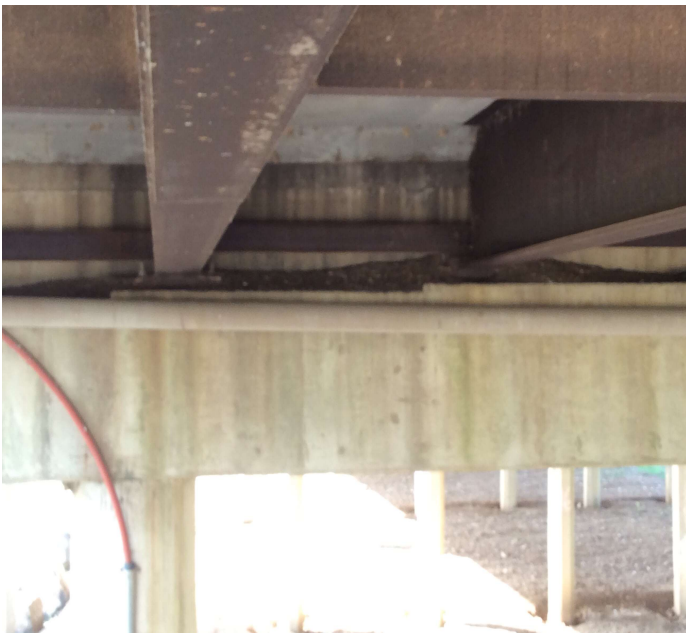
PHOTO 1 Description Debris on cap @ Bent 17.
