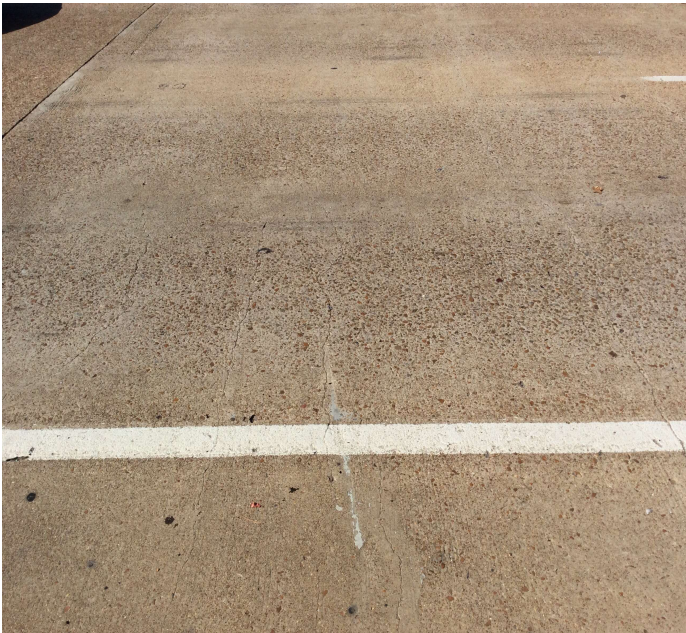
PHOTO 1 Description Transverse cracking to deck @ Span 23.
