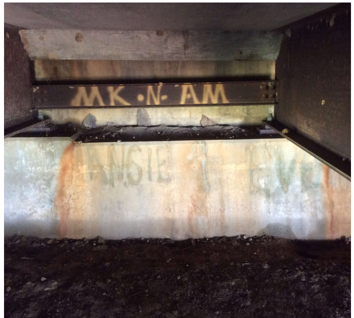
PHOTO 2 Description Debris on cap @ Abutment 2.
