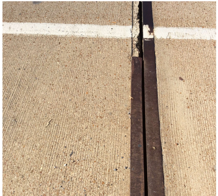
PHOTO 2 Description Joint material at Bent 17 Joint has fallen out and is missing.
