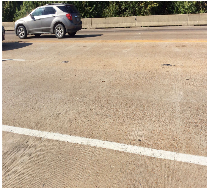
PHOTO 2 Description Transverse cracking to deck @ Span 20.
