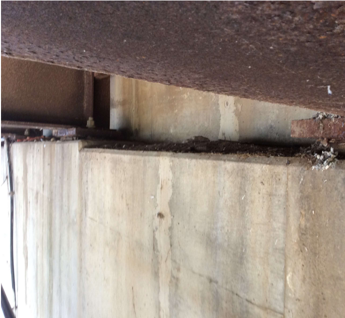
PHOTO 3 Description Debris on cap @ Bent 18.
