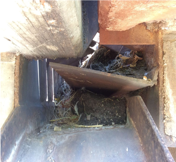
PHOTO 3 Description Debris in Finger joint @ Bent 18.
