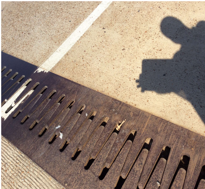
PHOTO 1 Description Debris in finger joint @ Bent 23.
