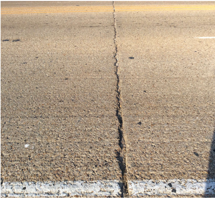
PHOTO 1 Description Debris impaction @ Bent 2.
