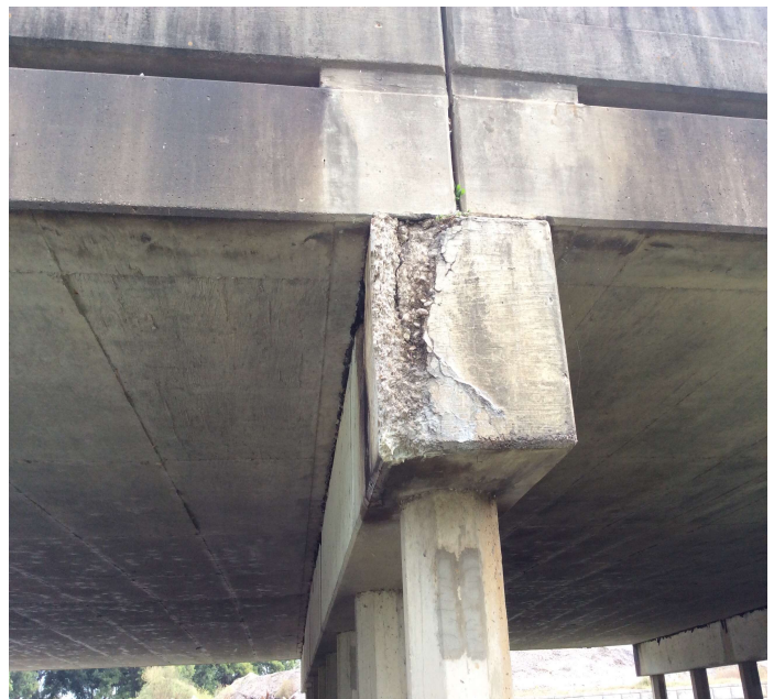
PHOTO 2 Description Large spall to Left end of cap @ Bent 3.
