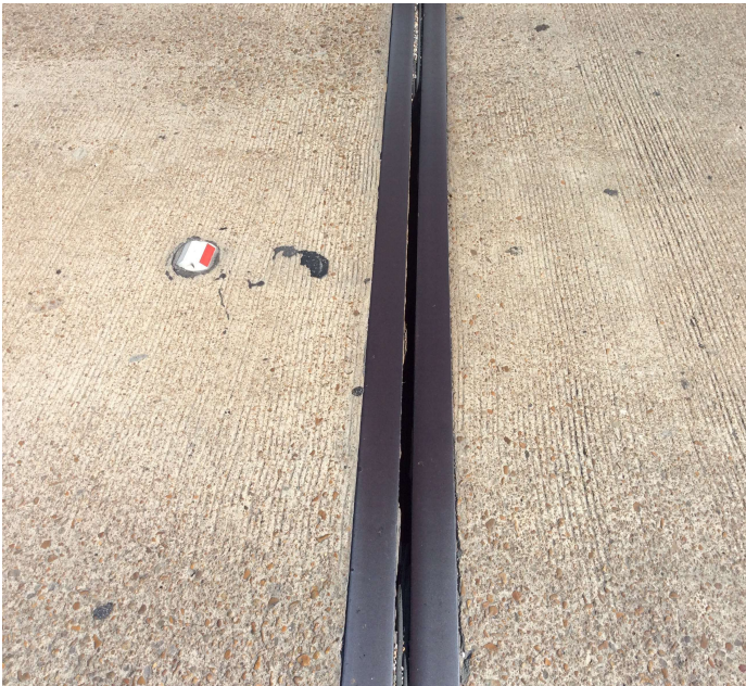
PHOTO 4 Description Joint material @ Bent 24 has fallen down @ is missing in Left lane.
